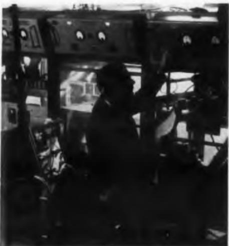
Eerie view at Sperry Gyroscope's Great Neck plant shows radar transmitter for the Army's Zeus anti-missile system under test. In the foreground is the high-power klystron; transmitter cabinets are in the background. Prior to shipment, the equipment is checked for output, stability and fidelity. The Army Ordnance Missile Command directs the development of Zeus, with Western Electric Co. as prime contractor.
