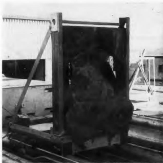
Fig. 1. In just over 1-1/2 hr, a hole was melted through this 1-in. lead shield by gamma flux of  $2 \times 10^{13}$  n/cm<sup>2</sup>-sec.
