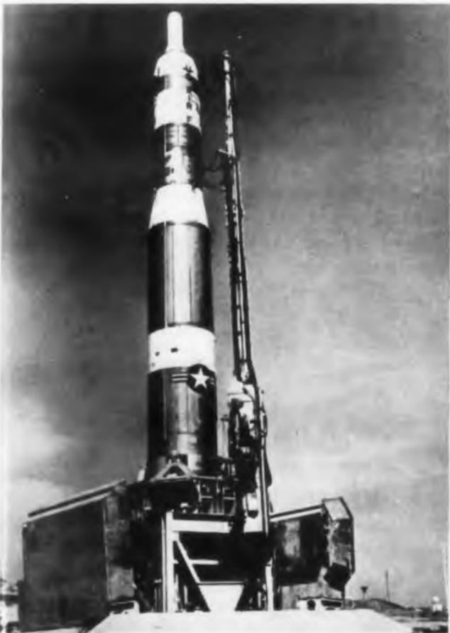
Titan ICBM check-out missile is in firing position in the underground launcher designed and built by American Machine & Foundry Co. of New York. The missile is fueled and guided from the underground launching complex. During the last few minutes of the countdown the doors open and the missile raised to ground level for launching.
