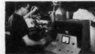
Helium mass spectrometer leak test performed on critical hermetic seal problems can detect a leak that would pass only 1 oz. of fluid in 500 years! Just one of 142 separate quality checks performed to make Gremar RF Connectors specified for use in all major missile programs.
