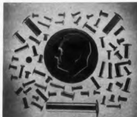
Designed for electronic and instrument uses, these rivets have 24-carat gold shot-burnished finish and are offered in range of lengths varying in fractional increments of 1/32 in. and in a range of diameters down to 1/32 in. The head form is a modified brazier with low contour and minimum functional diameter for the stresses imposed. Non-magnetic brass is used with the alloy controlled for ease in setting and uniformity of the swaged or upset clinch.
