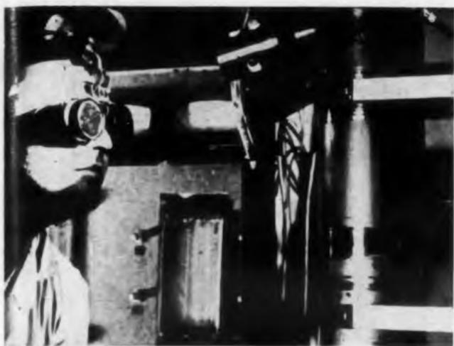
The new large single crystals are produced by the arc fusion process in individual furnaces like the one pictured here.
