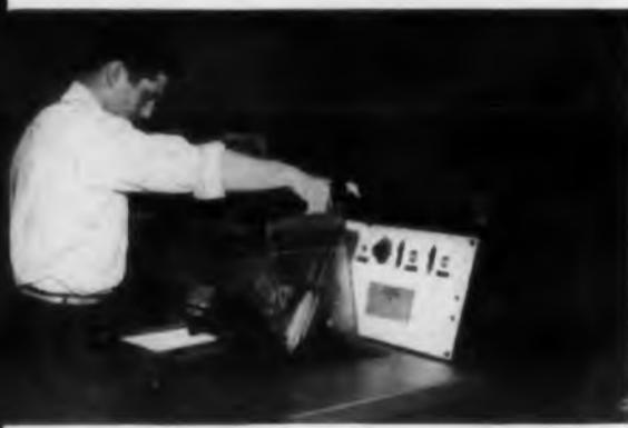
One of 3 Sel-Rex Platers in which Glass-Tite "barrel-plates" over 1-million components a week with Autronex Acid Gold.
