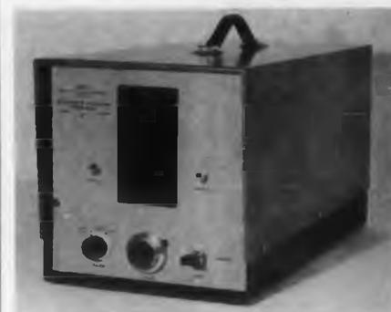
The Type 33-110 "Sadie" Digital Voltmeter has a sensitivity such that 100mv provides full-scale digital output (999). Controls permit selection of any voltage in either of two ranges
