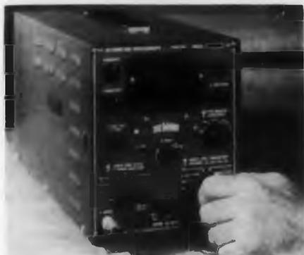
This cathode-ray oscillograph, Type 331, is particularly suited for field or laboratory testing and servicing of many types of electronic computers, as well as a variety of other equipment. The instru-
