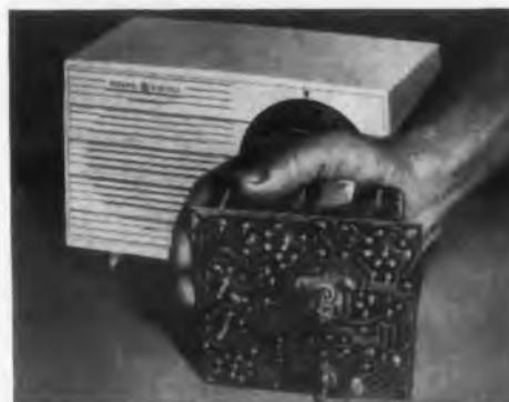
**COMPACT, LOW COST RADIO.** G-E Thru-Con Board permits compact chassis which slips into cabinet and plugs into speaker. Printed circuitry permits savings—cuts retail cost.
