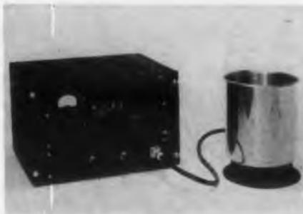
Consisting of a 1-gal capacity transducer driven by an ultrasonic generator, the Mixer - Cleaner Model 1115 is useful for such diverse applications as blind-hole clean-
