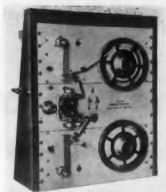
With start and stop times of 5millisec and tape speeds up to 60ips, the Model 903 Perforated Tape Handler offers character read-out of 150, 300, or 600 per sec.
