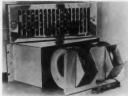
The Model 2E-408 Cabinet Cooling Fan is specially designed to fit the standard 19" electronic rack. It pressurizes the cabinet with filtered air, preventing dust from entering
