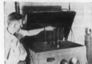
Control of metal finishes are a must for accurate relay operation. Parts are periodically subjected to a minimum 20% salt spray to check their resistance to corrosion.
