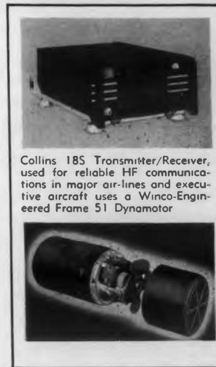
Collins 185 Transmitter/Receiver, used for reliable HF communications in major air-lines and executive aircraft uses a Winco-Engineered Frame 51 Dynamotor
