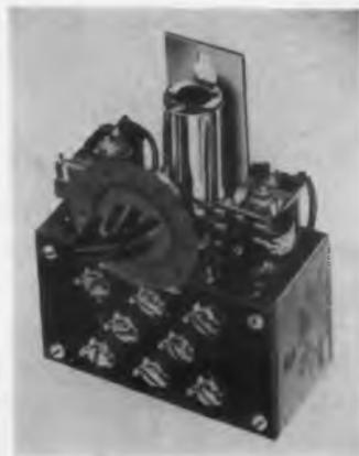
A repetitive series of circuit closures can be produced automatically by the Model S44 cold-cathode - tube electronic timer. The load circuit remains closed for a fixed time of about 60millisec, and the time between circuit closures can be adjusted to any value from as low as 0.03sec to 24sec.
