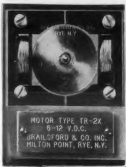
**Fig. 4. An experimental model of the transistor motor.**
