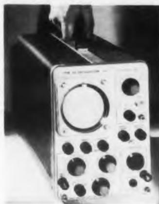
The Type 310 Oscilloscope is a d-c to 4Mc portable precision instrument, designed for both field and laboratory applications. With its small size (10" x 6-3/4" x 17") and light weight (23-1/2 lb) it is easily handled and fits into tight spots, yet is fully capable of handling many laboratory applications.
