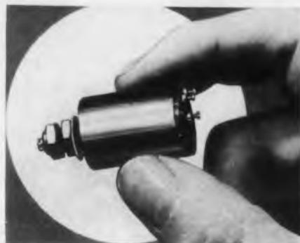
This 3/4" diam wire-wound potentiometer is available in standard values of 25, 500, 1000, 5000, 10,000, 50,000, and 100,000 ohms. A 5% resistance tolerance is standard with a temperature
