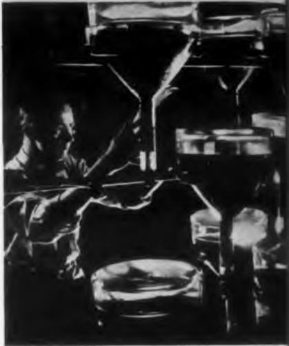
Coat inside walls of CRTs with a dispersion of 'dag' Colloidal Graphite in de-ionized water to retard secondary emission and adsorb gases. The resulting film also acts as an electric conductor and a ray-focusing material.
