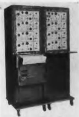
The eight-channel system is comprised of two units: a mobile cabinet containing an eight-channel recorder, control panel, and four driver amplifiers with power supplies; and a second mobile cabinet containing four additional driver amplifiers with power supplies, a sliding shelf, and cabinet space. The six-channel system is similar to the eight, but with fewer galvanometers, driver amplifiers, and power supplies. Sanborn Co., Industrial Div., Dept. ED, 195 Massachusetts Ave., Cambridge, Mass.
