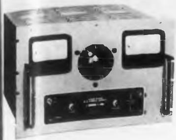
Model KM88 Aircraft Battery Eliminator is for testing and operating aircraft electrical and communication equipment. It operates on 115v a-c 60cy single phase and
