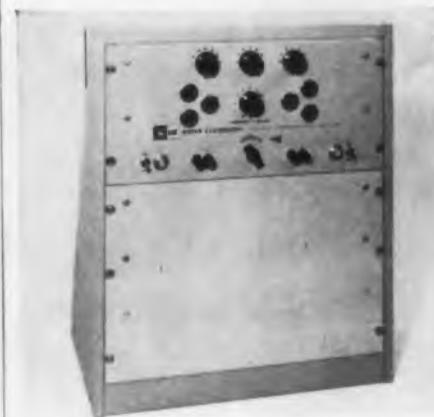
Meter Calibrator Model M100A-2 is a standard de reference that provides both voltage and current calibration range from 0 to 1000v and 200ma max, and from 0 to 100ma at 1000v max. The unit maintains long time stability
