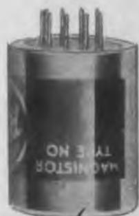
Amplification as well as information storage are applications for an unusual new ferroceramic element known as a "Magnistor". Shown at the left in actual size, these units can perform many of the functions of electron tubes, transistors, and other magnetic core devices. As amplifiers they have power gains up in the thousands. As memory units they can retain information indefinitely. Their life is long and not affected by temperature.
