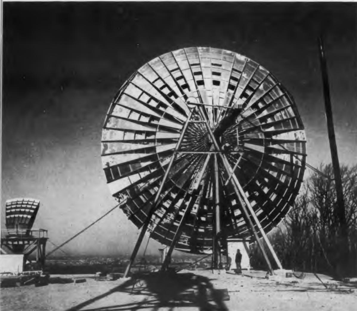
Over-the-horizon microwave transmission is accomplished with this 60' diameter experimental antenna. It has 30 times the surface area of the conventional antenna at left.
