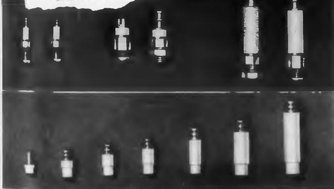
Illustrated are ERIE TEFLON STAND-OFF INSULATORS. The Erie-Chemelec Teflon line also includes Feed-Thru Insulators; seven and nine pin Miniature Tube Sockets in Teflon and Kel-F; Crystal Sockets; nine, fifteen and eighteen pin connectors, and five sizes of spaghetti in three colors.
