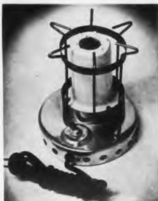
The "Horo" Electro-Bunsen Burner, is capable of achieving temperatures of 850°C under continuous operation, yet eliminates the hazard of fire and explosion. Operation is clean and odorless, because heating is accomplished by a stream of hot air, and no soot is deposited on the heated object. Heat is even, with no local over-
