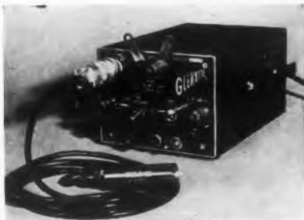
The "Glennite" F 408 decade amplifier is designed for general laboratory use and is provided with an input cathode follower probe. The probe is mounted on a 9'
