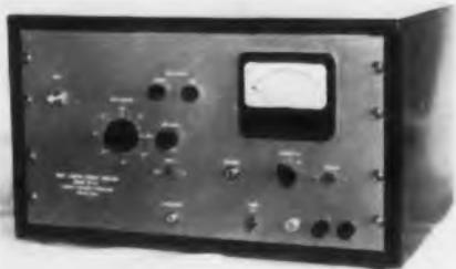
The Model D-C 151 Milli-Micro-Microammeter is an a-c operated instrument for measurement of d-c from  $3 \times 10^{-15}$  amp to  $10^{-7}$  amp. The
