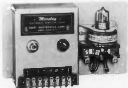
The "Micrelay" is designed for control of high-power, high-current loads up to 60amp or 3hp from very low-current, low-power devices or circuits. Typical activating devices are: photocells; thermostats and other thermal instruments; meter-type contacts; and circuits controlled by resistivity of fluids and capacitance of dielectrics.
