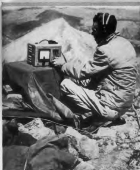
Taking antenna field strength readings atop 13,783 ft. Mt. McNamee.
