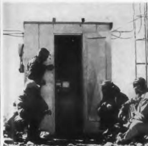
Installation crew watching the first TV reception on test equipment in the amplifier shack. In normal operation, the insulated 6' x 6' metal building houses the front end amplifier equipment for the community antenna system.
