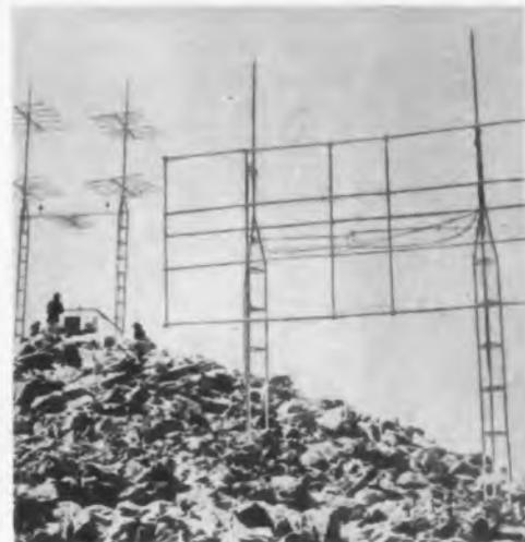
Two antenna groups receive channels 2, 4, 7, and 9 from Denver stations, about 60 air miles away. The first antennas suffered considerable damage from icing and high winds, and had to be replaced with sturdier structures. The coaxial cables however, insulated with BAKELITE Polyethylene and jacketed with BAKELITE Vinyl Plastic, measured up to expectations from the very first. Note the loose, broken rock, typical of the terrain along the course of the primary lead cable.
