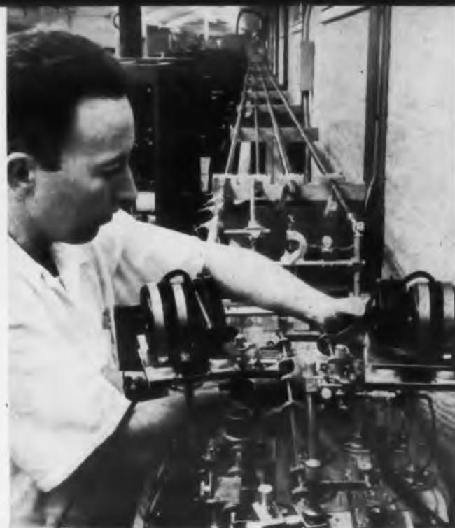
This Bell Telephone Laboratories engineer is testing various long-distance waveguides to determine the optimum diameter.
