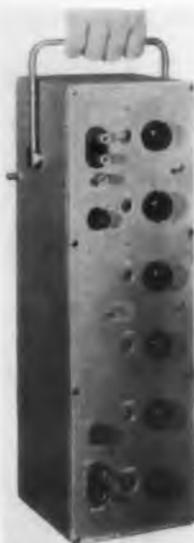
Two new versions of the "Standard Ratio Transformer" (a-c voltage divider) are available. Both models permit rapid selection of accurate voltage ratios by means of rotary switches. Five decade switches, followed by a single-turn potentiometer, provide continuous resolution and readout of better than six significant figures. Ratio value is indicated as direct decimal reading. Every switch position displays its corresponding digit through a dust-proof window.
