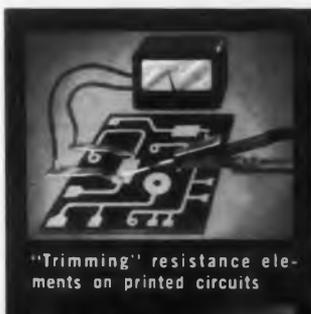
"Trimming" resistance elements on printed circuits
