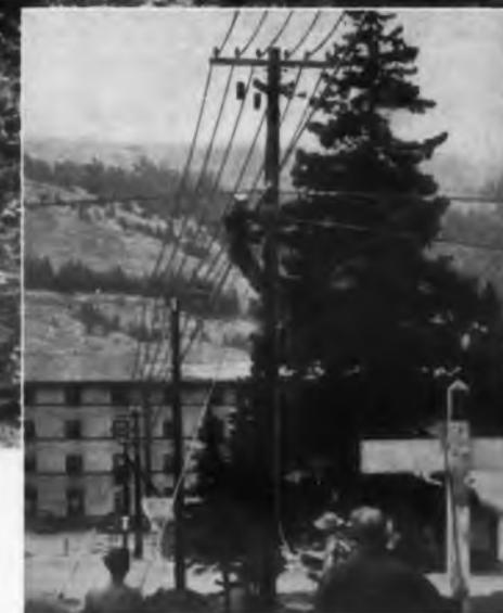
Stringing RG-11U cable on existing telephone poles. RG-11U was used as secondary lead, and as drop cable to individual outlets.
