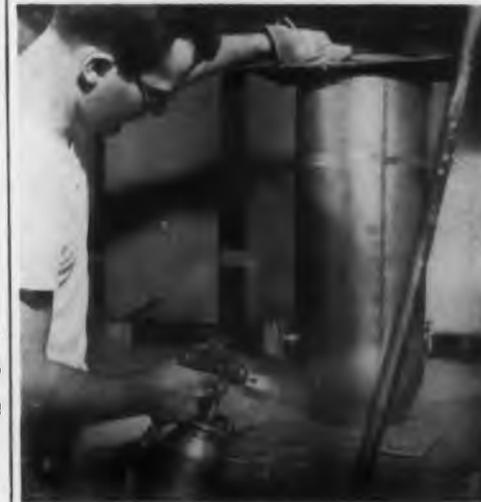
After a one hour bake at 400 F, the silicone based coating provides the required protection. According to Solar, this is one of the most satisfactory paints for use on jet engine parts. No. 28
