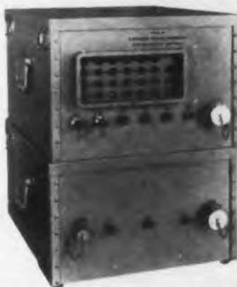
The 8Mc Counter Chronograph, Model 471, is a rugged instrument for testing radar and sonar equipment. It is designed to permit calibration and other detailed tests under field or shipboard conditions. Housed in two drip-proof heavy-gage reinforced aluminum cabinets, it contains
