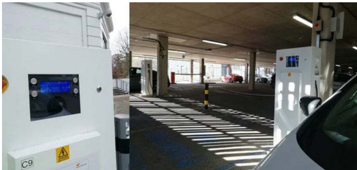
These bidirectional EV charging units were developed as part of the VIGIL project operating on-site at Aston University.
