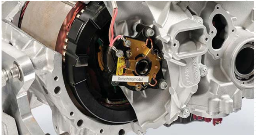
3. Shown is a close-up of the slip-ring assembly that powers the rotor of the motor used in BMW's iX-M60 electric SUV. BMW
