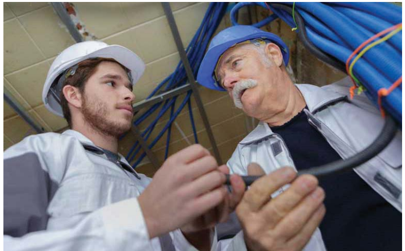
2. The performance of the cabling and interconnects are related to the safety of the facility and its operators. Image: Auremar 160939515 | Dreamstime
