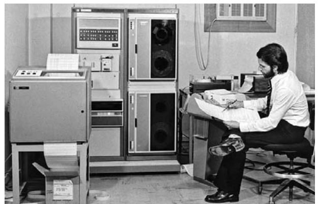
4. The 16-bit HP 2100 minicomputer had 16 kB of magnetic core memory and used magnetic tape for removable storage. (Courtesy of Creative Commons)
