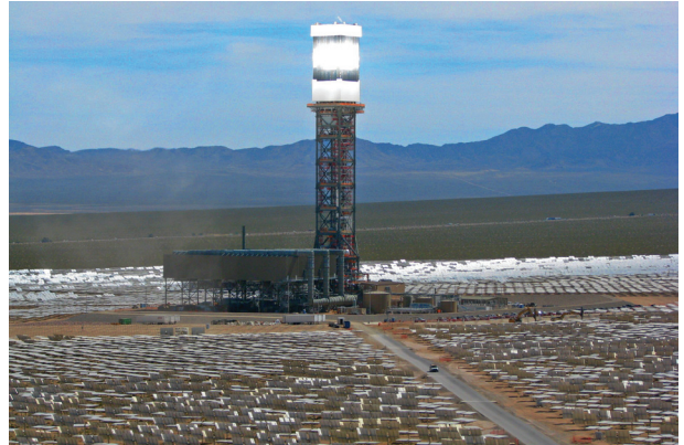
IoT Technologies can coordinate the rotation of the hundreds of thousands of mirrors to maximize energy production at the Ivanpah Solar Electric Generating System on the California-Nevada border. (courtesy of Business Wire)
