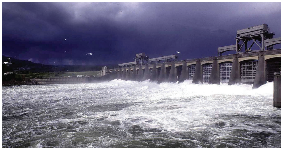
1. Bonneville Dam is roughly 200 feet high and half a mile long as it spans the Columbia River. Its 20 turbine-powered generators have a combined capacity of 1.189 GW. They literally “don’t build them like that anymore.” There isn’t room. Load management addresses that limitation, but engineers also are dealing with an accumulated legacy of systems and processes that present daunting prospects for creating feedback systems that will work at this scale. (courtesy of the Bonneville Power Administration)
