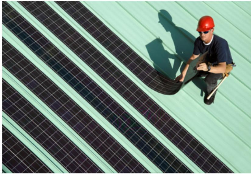
5. Lighter than c-Si panels, SoloPower's flexible thin-film solar panels install easily on commercial rooftops.
